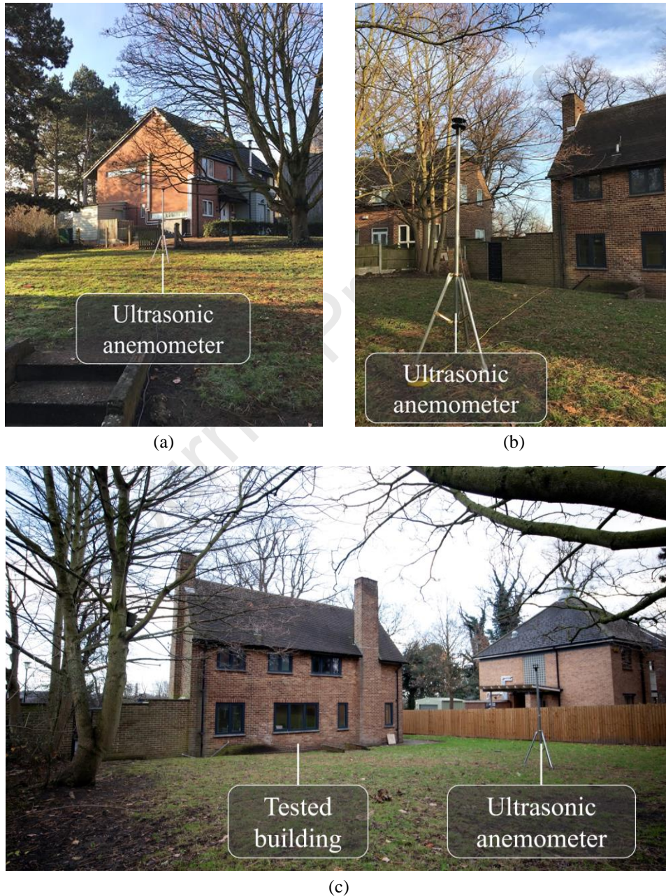
Figure 8: Photos of surrounding environment of the installed ultrasonic anemometer
