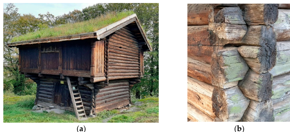
Figure 3. (a) A heritage log house building in Tønsberg, Norway. (b) Carpentry corner joint of the logs.
