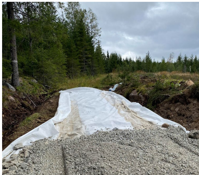
Figure 3-1: Geotex 2000 landscape fabric made of polypropylene here used for erosion control when constructing new roads in Finnskogen, Norway (photo credit: private).
