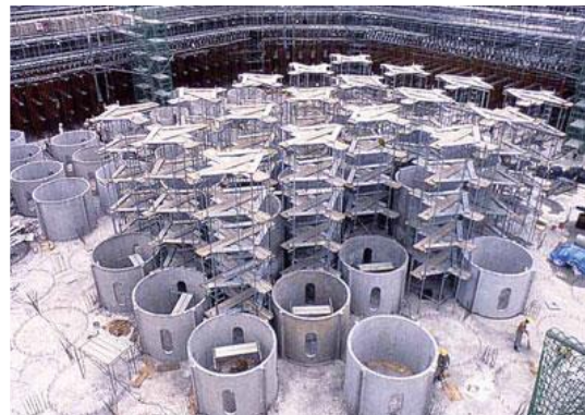
(b) Honeycomb construction (Wang, 2015)
