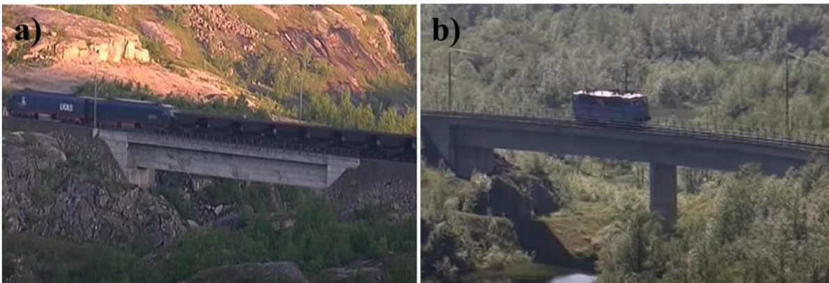
Figure 15. Different trains crossing the bridges; a) Iron ore train, b) Lightweight railway vehicle.
