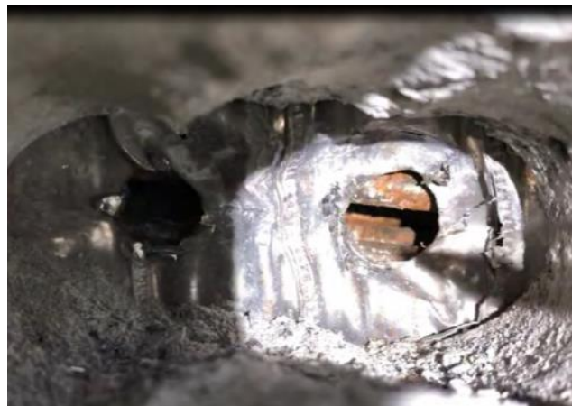
Figure 66 Drilling and visual check of 3SC [76]
