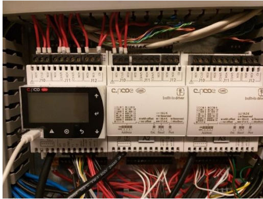
Figur 19: Carel PLS; c.pCO mini high end + 2stk c.pCo extension
