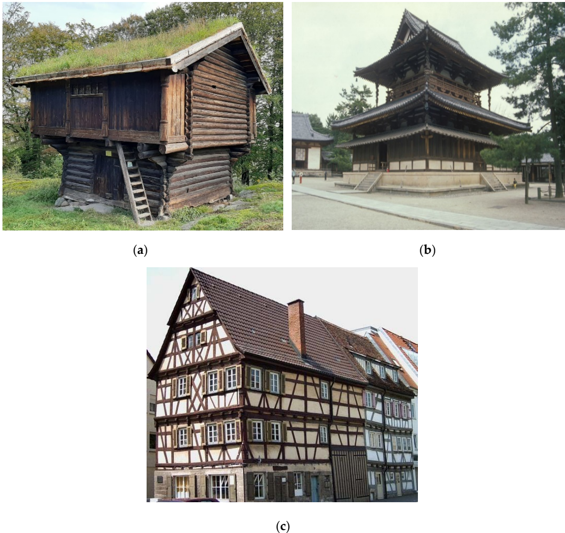
Figure 3. (a) Log house (Heierstad Loft, Tønsberg, Norway); (b) Post and beam (The Golden Hall (Kondo) of the Horyu-ji Buddhist temple, Nara, Japan) reprinted from [4]; (c) Timber frame building (Baden-Württemberg, Germany) reprinted from [19].
