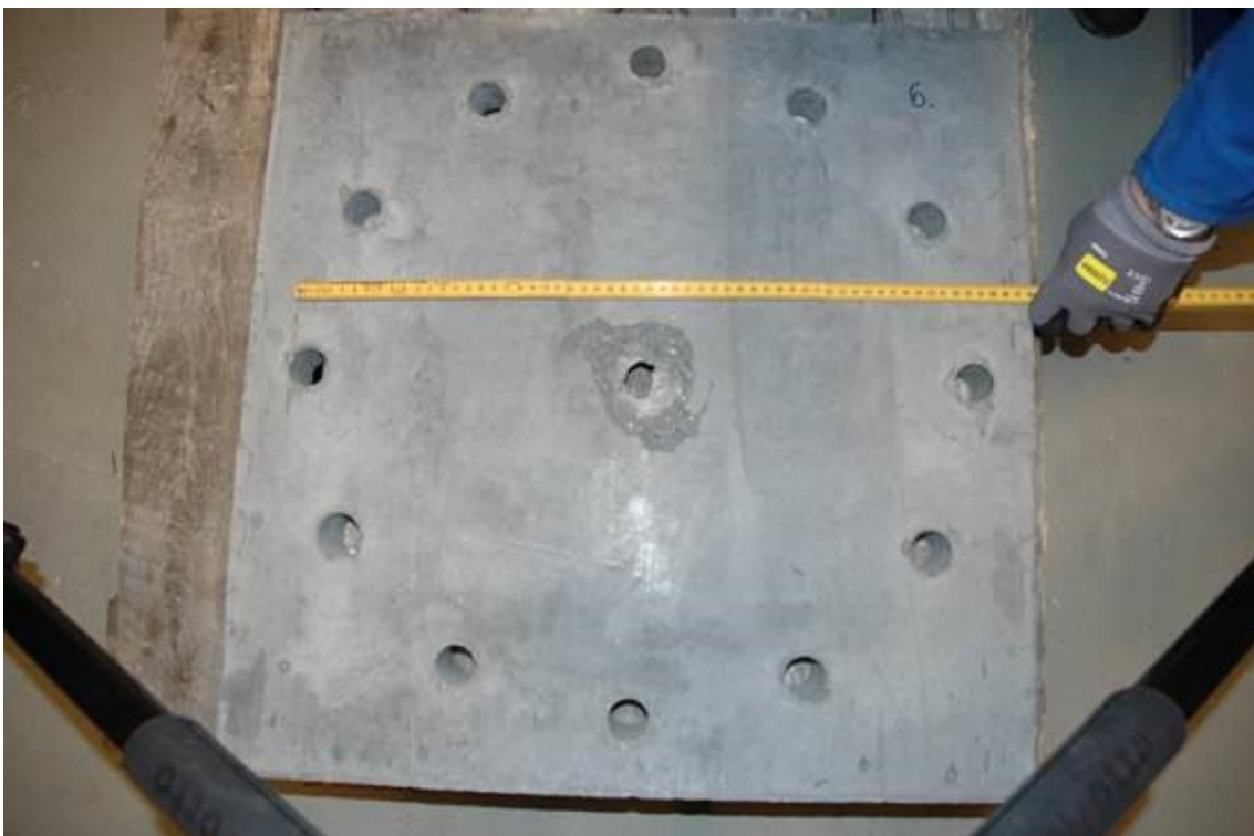
Figure 24: Spalling from test 6 with concrete C110
