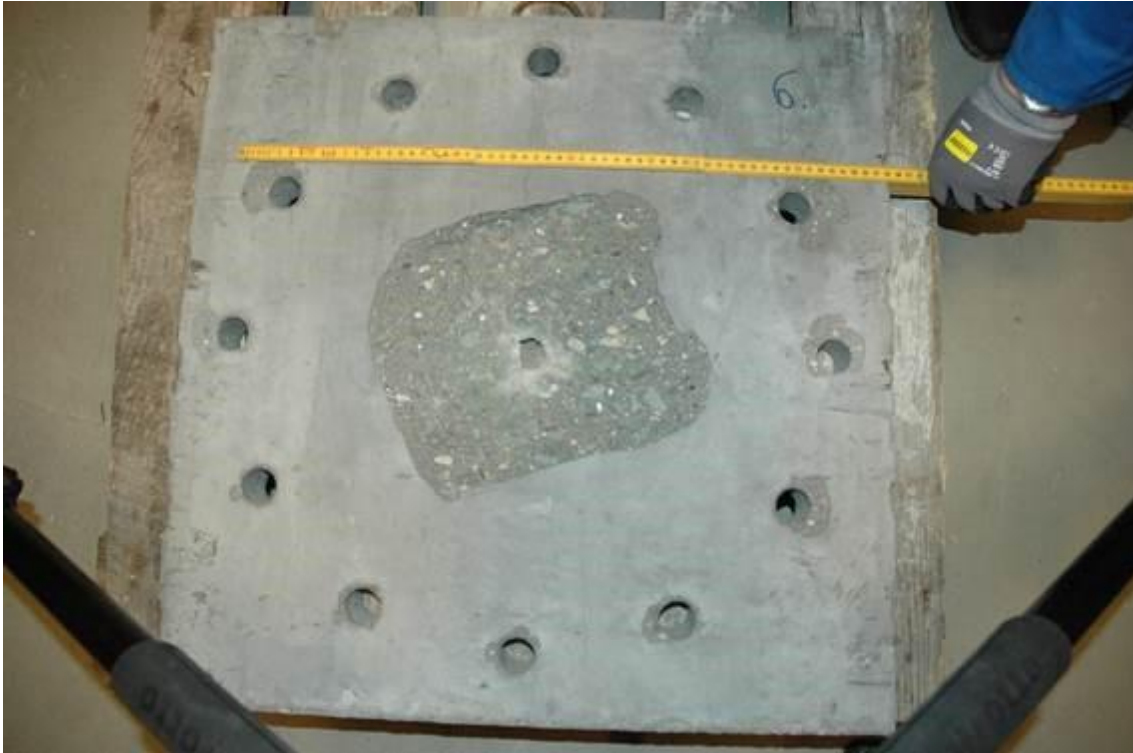
Figure 25: Scabbing from test 6 with concrete C110
