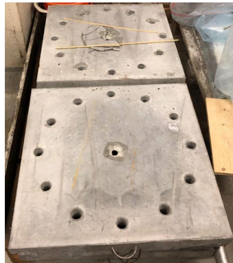
Figure 23: Perforated concrete plates.
