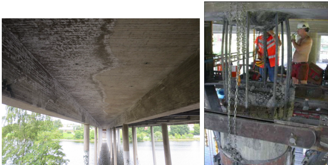
Figure 2.26: ASR consequences on Elgeseter bridge [21]
