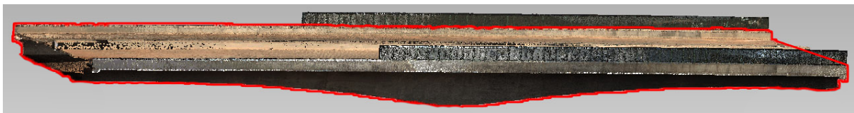
Figure 3.9: Highlighted superstructure of the Dade Bridge
