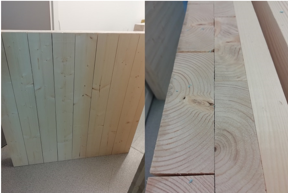
Figure 20: Solid timber element from Norsk Massivtre
