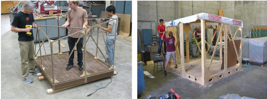
Figure 4. Version 1 (left) was built of composite material at half-scale; Version 2 (right) was explored at full-scale using wood products.
