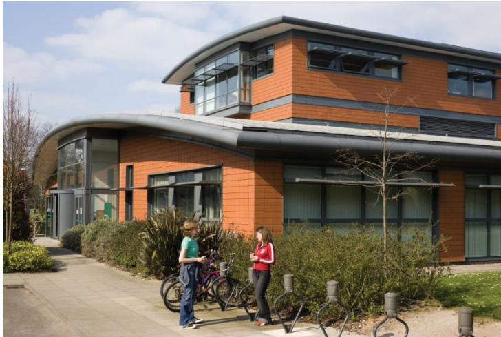
Figure 4. Survey 'Campus Image C' (University of Nottingham Sutton Bonnington campus Plant Sciences building). Source: University of Nottingham image bank, Martine Hamilton Knight Photography, 2009.
