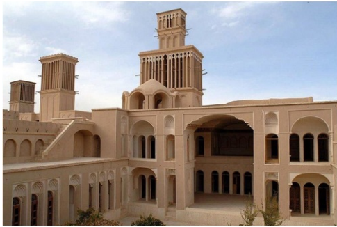
Fig. 1 Natural cooling using double wind tower and cistern in a traditional building in Yazd (Iran).
