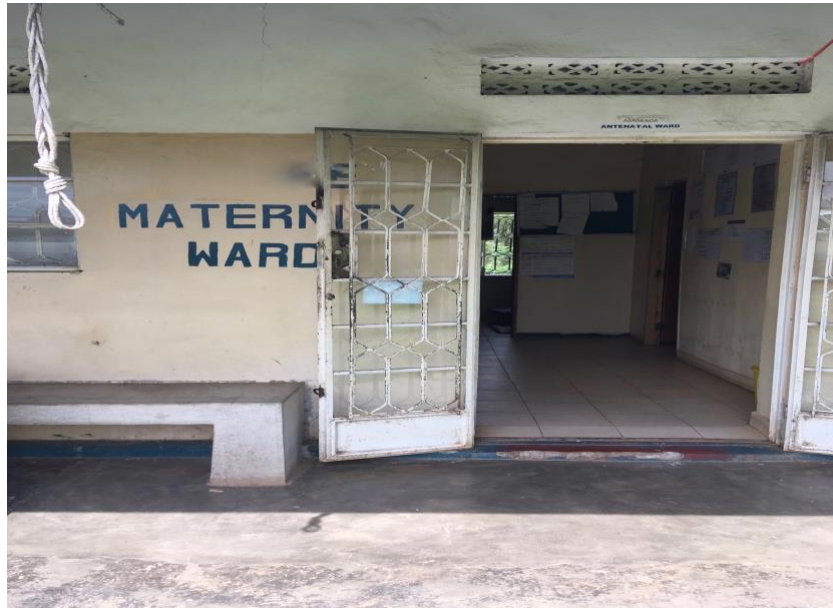
Figure 4 HCIII Maternity Ward
