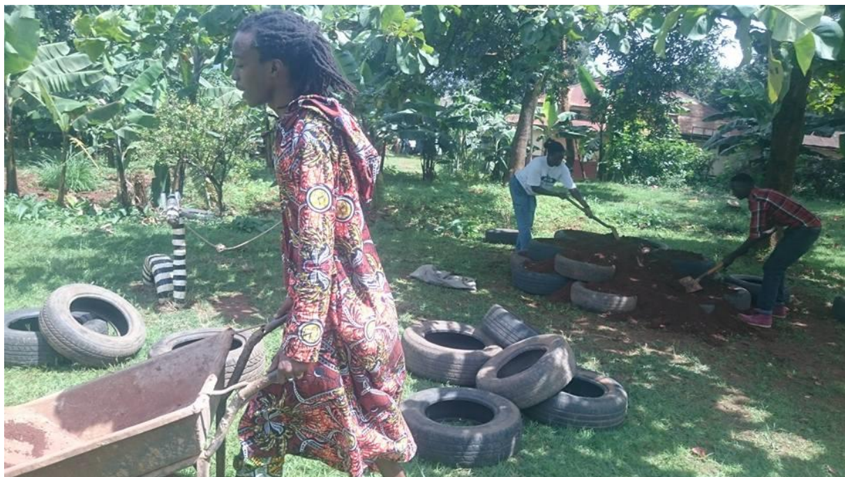
PICTURE 18: Artists carrying car tires to the playground construction site.
