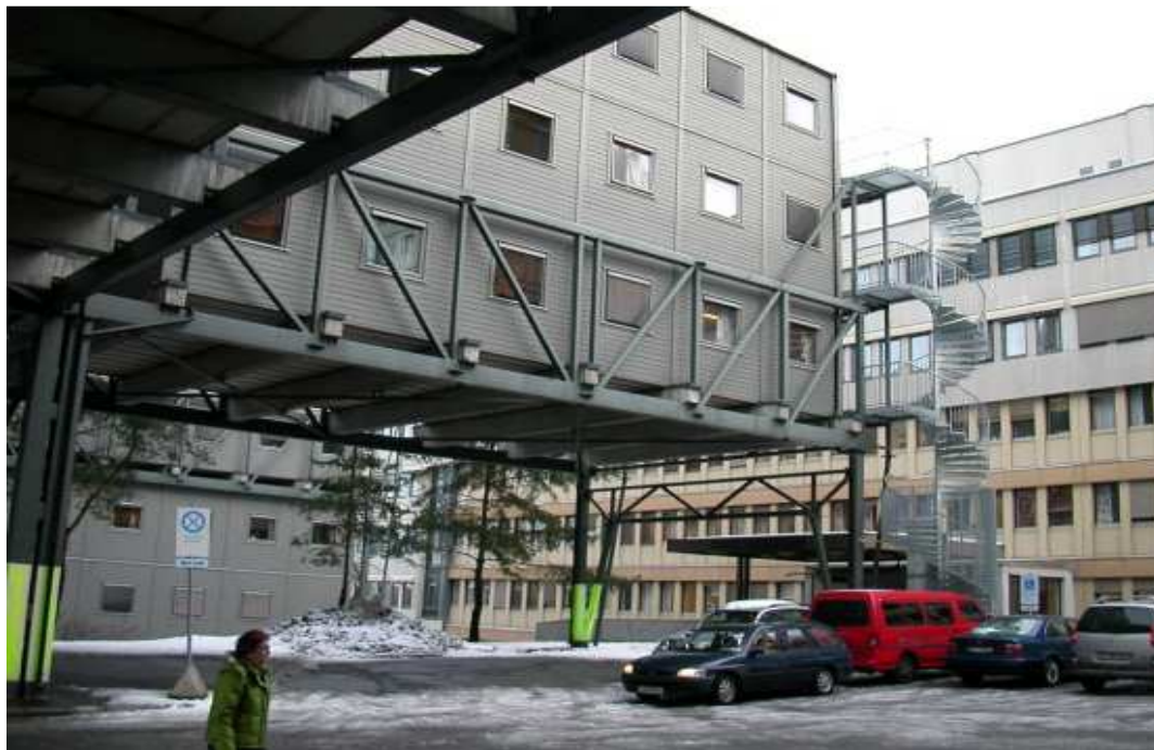
Picture 2: External hospital façades of Akershus University Hospital – the old hospital was being rebuilt in 2010 (Lørenskog).
